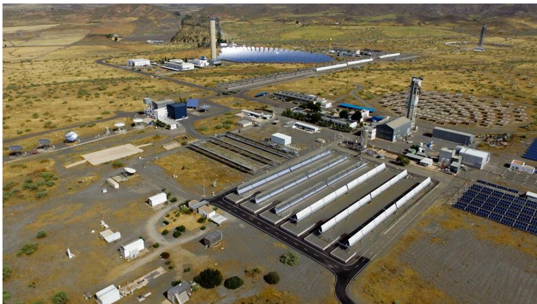
Figure 2. Aerial view of the PSA
