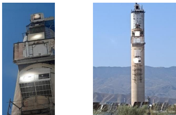
Figure 18. THICAV receiver prototype at the CESA-1 tower: (left) detailed view of the receiver panel installed on the tower; (right) general view of the CESA-1 tower during the test campaign.
