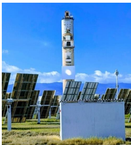
Figure 60. The CESA-I facility seen from the north.
