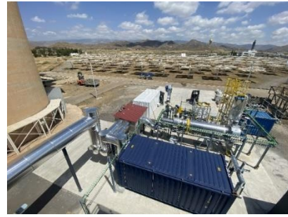
Figure 19. Right: Odqa's air-based receiver inside the CESA-1 tower. Left: Odqa's high temperature CST industrial demonstration system
